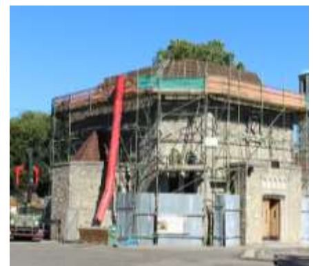
Work on St Joseph's chapel roof is progressing well
